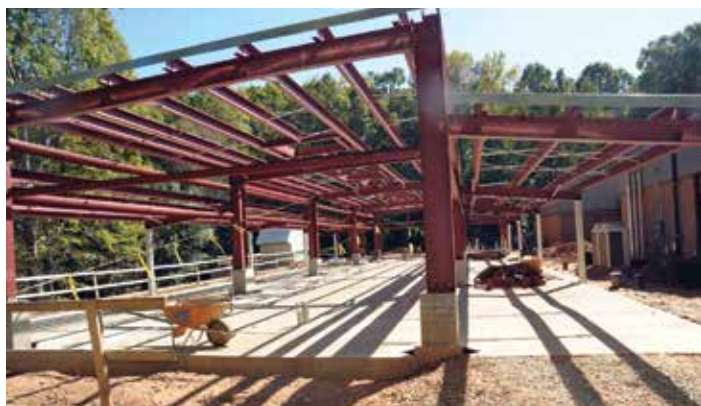
Weather permitting, November 18 is the target completion date for Phase I, the construction of a 5,500-square-foot structure that will replace the aging kennel next to Halbert Hall with an expanded housing and learning facility.
